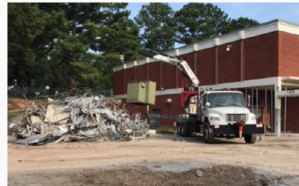
Georgia Power transformer removal
